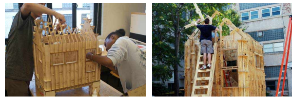
Figure 6 Laser cut model at 1'' = 1'-0'' (a), the same information used to build the final house (b) constructed exclusively of \frac{3}{4}'' plywood with studs and furniture.
