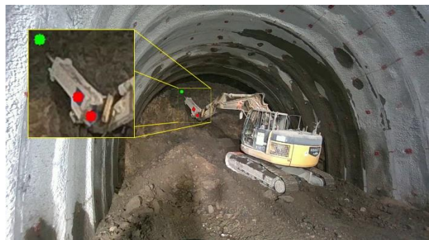
Figure. 9 Marker detection and excavation point using Fig. 6
