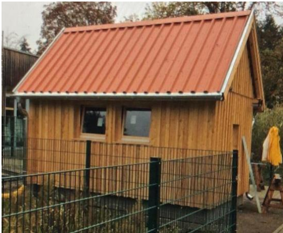
Figure 20: Smart Energy House in Berlin (Germany).
