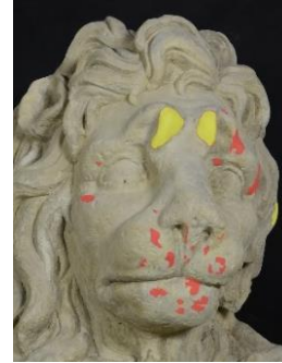
Figure 3: The loss compensation methods: Yellow: insertion of replacement stone, Red: composite repairs (Photograph by Anna Duda-Maczuga)
