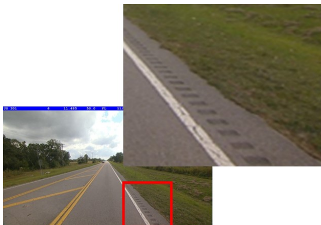
Figure 3 Example of shoulder rumble strip
