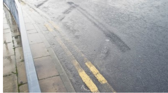
Figure 5: A worn out yellow double line is depicted on a wet road surface [10], that can be detected by machine vision using contrast and color separation features
