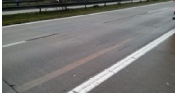
Figure 4: In this figure a set of standard white lane markers are shown next to a set of yellow lane markers [9]. Depending on the context either of the two types of lane markers is the guiding one, and thus both needs to be detected. A contrast detection of the luminance difference between marker and background is necessary as well as a color separation of the yellow against the white marking.
