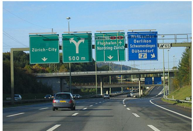
Figure 12: In Switzerland Freeway traffic signs are green and signs for highways are blue.
