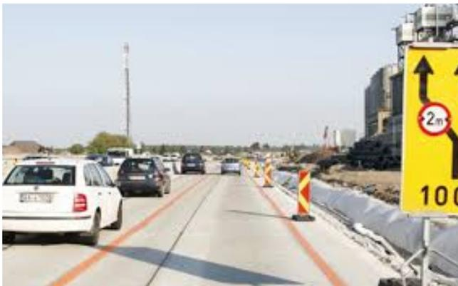
Figure 10: In Austria construction zone lane markers are orange.
