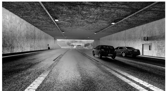
Figure 7: Tunnel exit, captured and correctly tone mapped with a camera with high dynamic range ability. The objects outside the tunnel are clearly visible.
