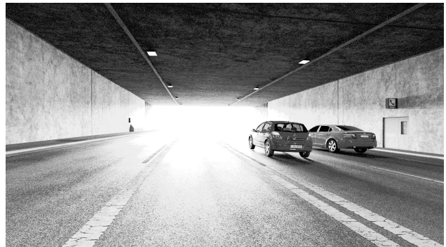
Figure 6: Tunnel exit, captured with a camera with limited dynamic range ability. The objects outside the tunnel are not visible.
