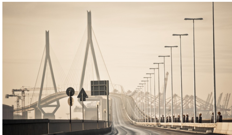
Figure 2: Eastern view of Köhlbrandbrücke in Hamburg (Germany). In the foreground, the eastern ramp can be seen. In the background is the cable-stayed bridge with 135 m high steel beams [4].
