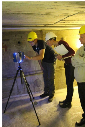
Figure 9: Setting up the 3D-LiDAR-Scanner for measurement in the hollow box girder.
