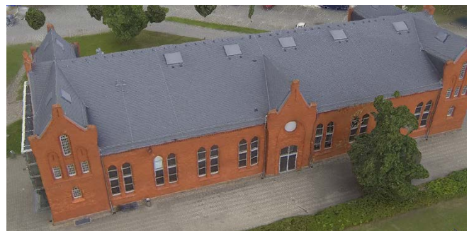
Figure 5. Reconstruction of the auditorium, textured mesh, without EXIF-data
