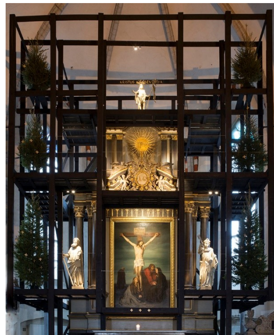
Figure 1. Specially designed and built long-term scaffoldings in front of the St. Mary's Cathedral's retable. Photo: A.Uueni, 2017
