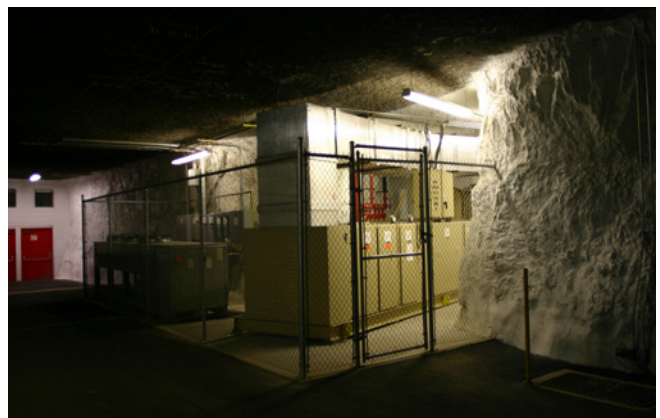
Refrigeration, dehumidification, and air-filtration systems are located outside the vault for non-disruptive servicing. The year-round 55°F (12.8°C) ambient temperature in the mine provides a steady-state environment for energy-efficient HVAC systems.
